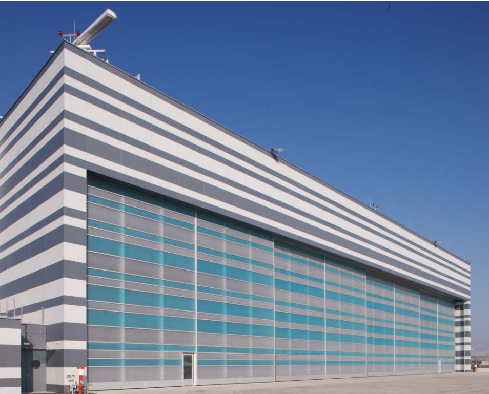
Translucent fibreglass creates pleasant lighting conditions in the hall.
